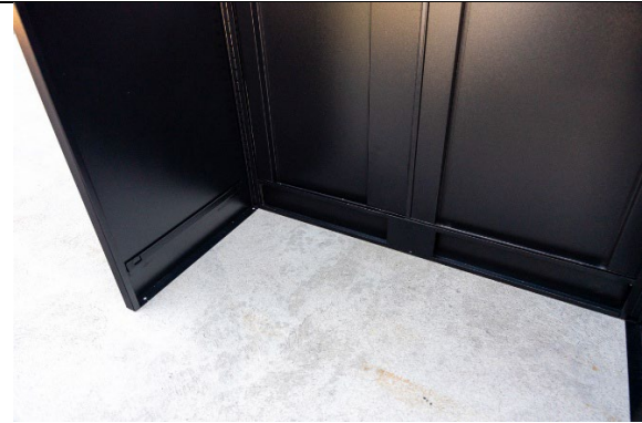
Fig. 17. Bottom corner of the right-side panel slotted to the door
