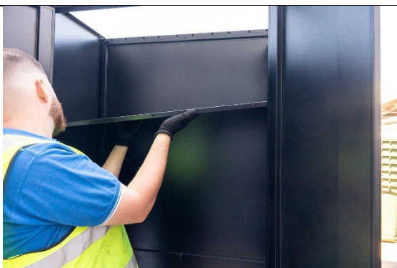
Fig. 25. The H flaps on the top panel should be facing you as you put it into place.
