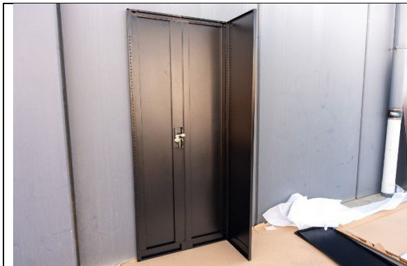
Fig. 8. Left side panel slotted into the door panel.
