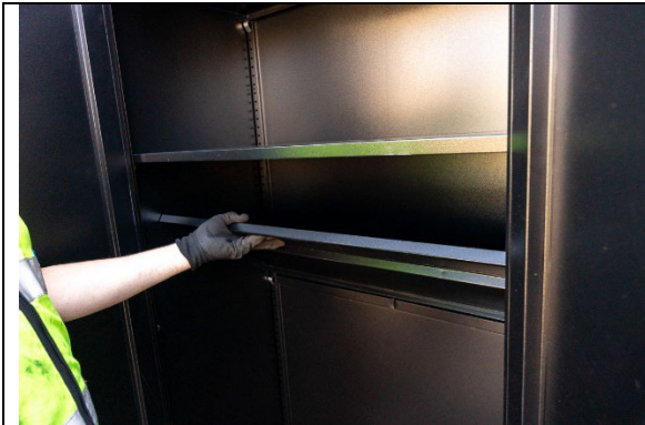
Fig. 38. Placing the shelves on the shelf supports.
